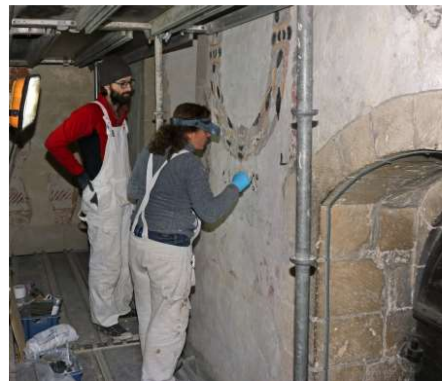
Claudia Fiocchi demonstrating paint reattachment techniques on the north wall (right)
