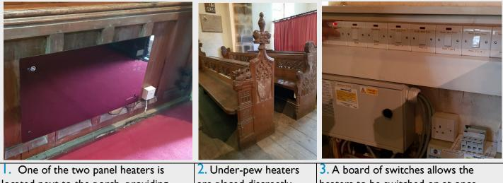
I. One of the two panel heaters is located next to the porch, providing warmth upon entry to the church. The other is fitted behind the altar. 2. Under-pew heaters are placed discreetly throughout the building. Here a switch can be made out on the choir stalls. 3. A board of switches allows the heaters to be switched on at once when needed. Additional switches on the heaters themselves allow for individuals to turn them off, if desired.
