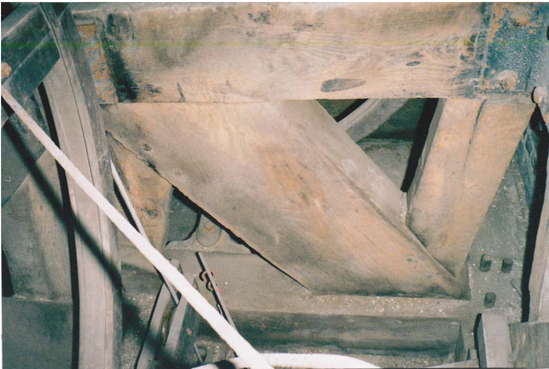
Typical use of a double jack-brace, on a massive brace at the south-west corner of the pit for the sixth bell.
