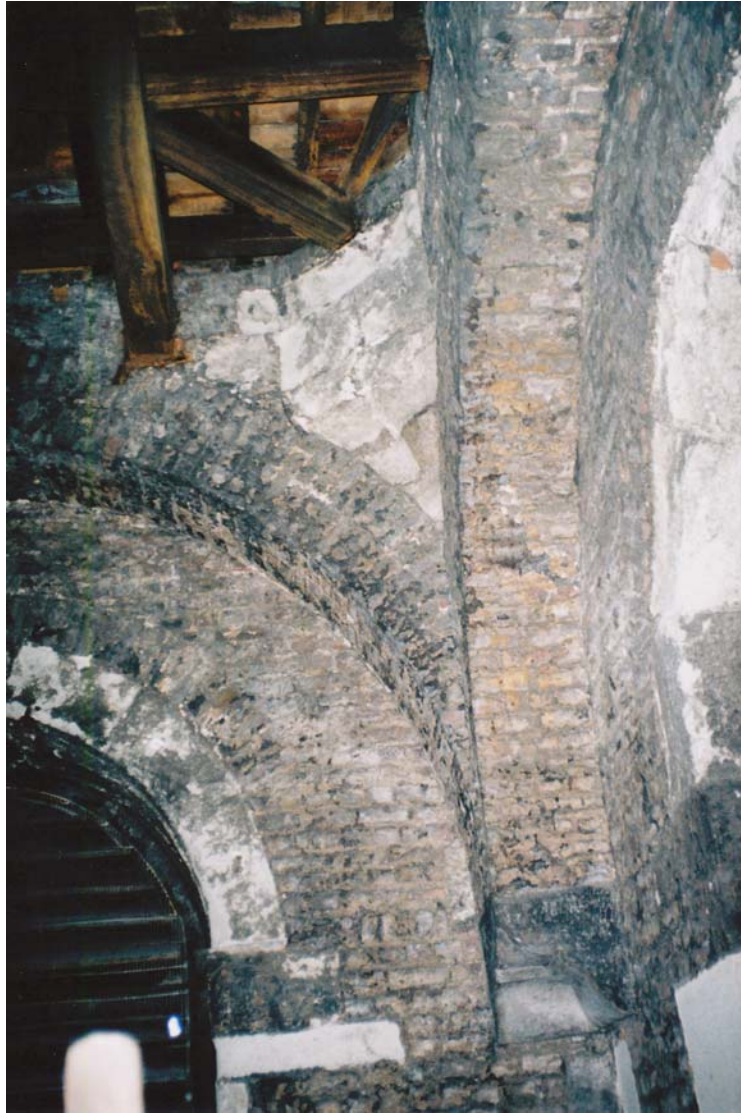
The squinches supporting the octagonal stage above the belfry.
