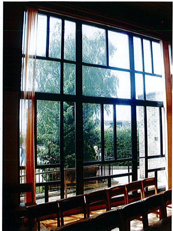
Photograph taken from the left hand side of the window.
