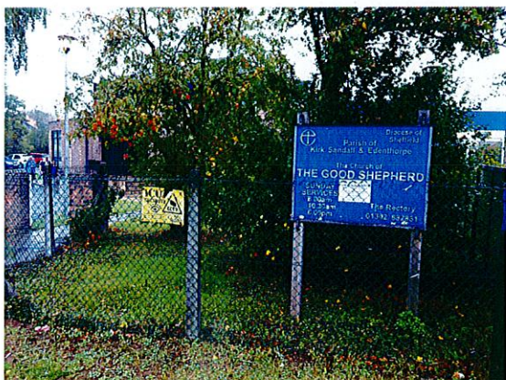
The chain-link and concrete post boundary and existing notice board, due for removal and replacement
