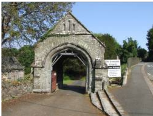
The lych-gate seen from the west, these temporary struts now removed
