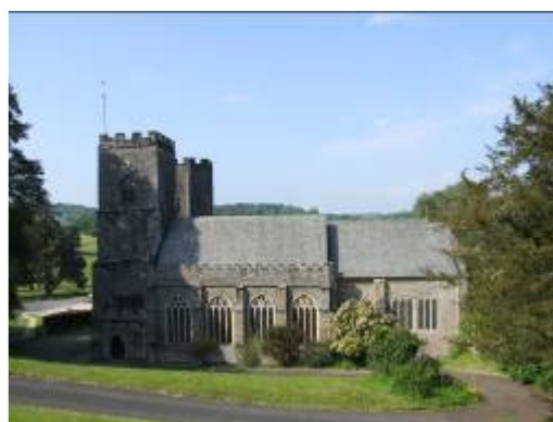
The church seen from the south
