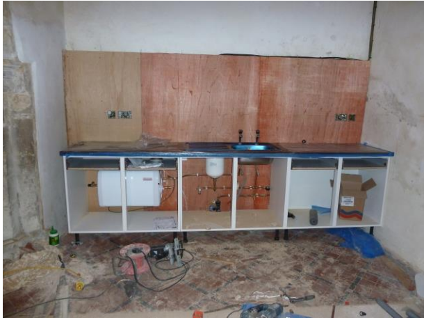
Kitchen, water heater and pipe work in position Kitchen complete with new boiling water unit
