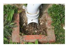
If the drainage system does not direct the rainwater away from the building it will lead to severe problems causing the instability of foundations and rising damp.
