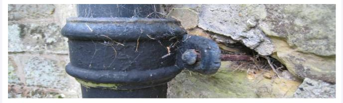
Rainwater goods include the gutters and downpipes which are key to the survival of a church building. Together with a watertight roof, they ensure that rainwater is directed safely away from the building.
