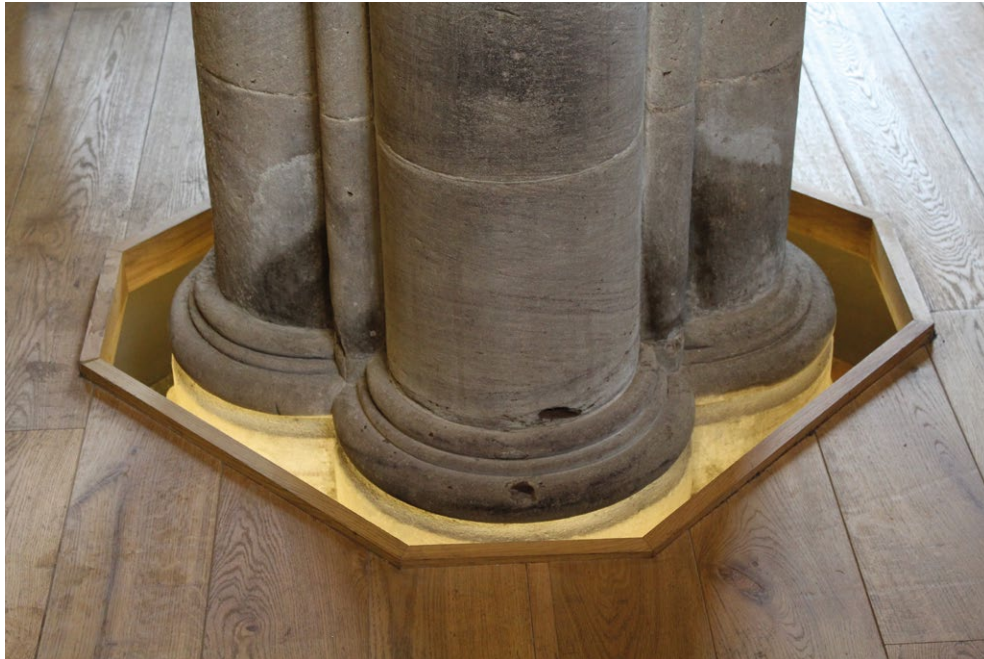
St Peter's, Hereford, design detail after floor was raised
