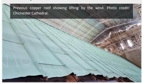
DBR Ltd were commissioned to undertake restoration works of the quire roof. Contractors visited the site in December 2017 and scaffolding was erected in preparation for the repair work in February 2018.
