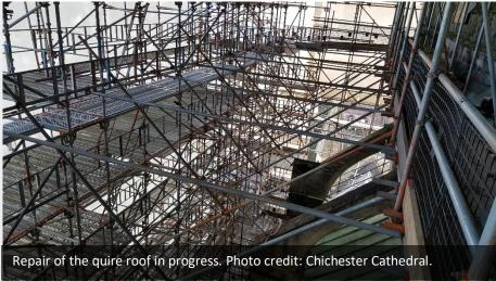
in concrete, and fire prevention measures in the 1990s, had exacerbated the problems by restricting air flows and inadvertently creating an environment conducive to damp, death watch beetle and timber decay. This was the first phase of a £4.9 million programme of works to the high roofs. The balance of the costs were met from fundraising by the Chichester Cathedral Restoration and Development Trust.
