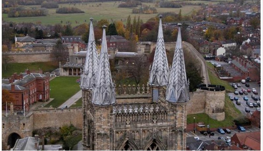
Four of the twelve pinnacles. Photo credit: Buttress Architects.
