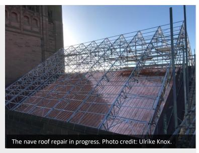
vibrations had allowed 'star fractures' to develop in the weakened copper panels, creating leaks, and there was also a risk of sections of roof flying away in the wind. A substantial area of roof was replaced in the early 1990s following storm damage, but its fixtures were failing. In addition there was widespread concrete deterioration to the cathedral's roof structure, partly caused by water leaking from the damaged roofs.
