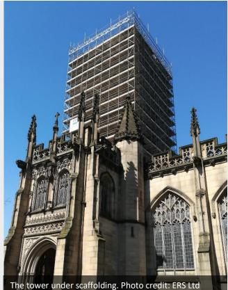
stone, louvres replacement and the removal of vegetation from the tower. The tower roof is also being replaced.
