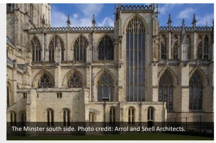
foreseeable future, as its magnesian limestone is prone to deterioration where exposed, and problems have been compounded by past repairs using stones of different geologies and the extensive use of wrought iron fixings which are now corroding, expanding and causing masonry to fail.
