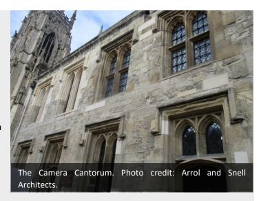
of Magnesian limestone which is particularly vulnerable to a variety of different decay mechanisms. There can also be difficulties with 19th-century construction arising from iron cramp damage or poor stone selection.
