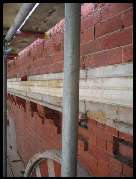
Ketton limestone cornice and parapet above recommended for replacement because it had reached the end of its 'serviceable life'
