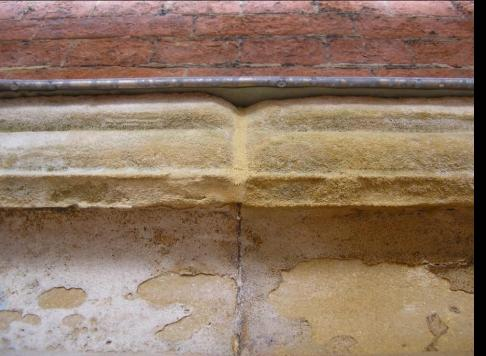
Refilling open and decayed mortar joints, limited masonry repair and installation of a lead weathering to reduce long term decay and maintenance
