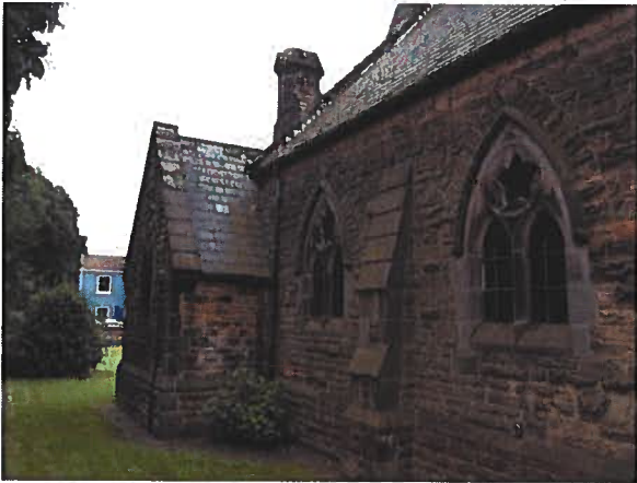
Nave and Vestry viewing from North
