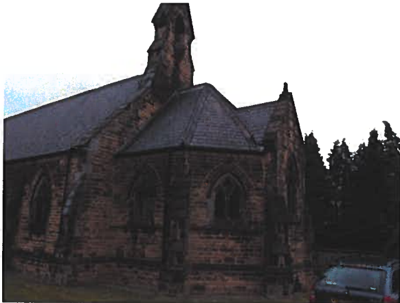
Chancel Apse from South East
