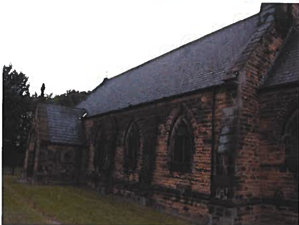
Nave South side
