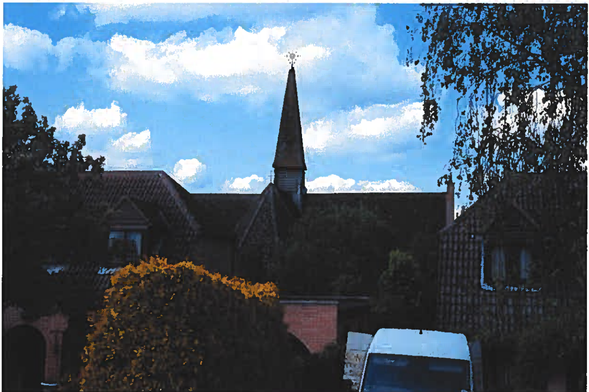
View of the Church from Padnal Bank at the North East
