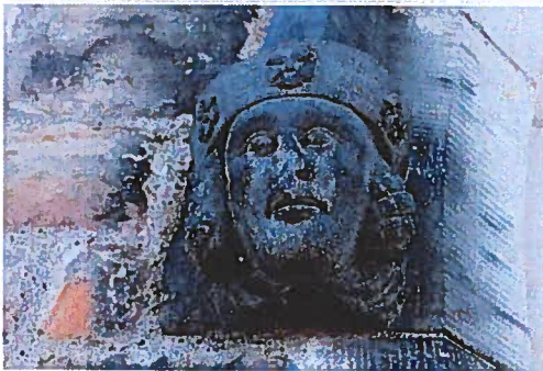
S Porch headstop (left)
