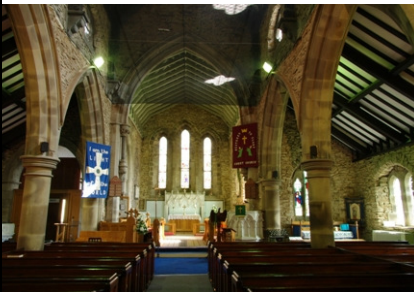
Interior view E
