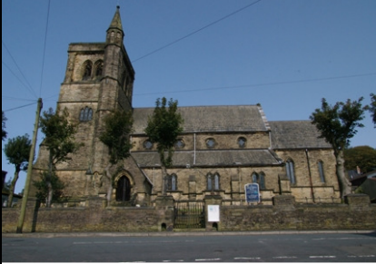
S elevation from Christ Church Street
