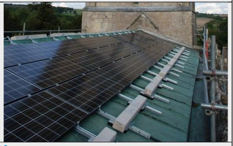
2 Clamping was not possible, so the solar panels are affixed to stainless steel Unistrut rails to which weights are clamped at each end. The solar panels contribute to St Michael's becoming a "net zero carbon" church.
