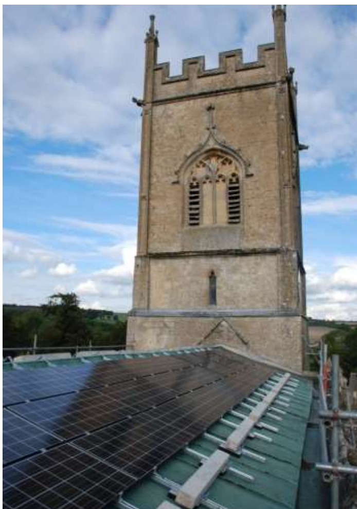
Left: Solar panels at Withington, St Michael and All Angels.
