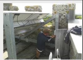
3 The panels were installed on the preexisting wind turbine frame, saving costs and avoiding further changes to the existing masonry.
