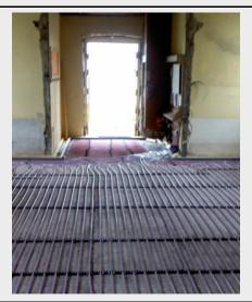
2 Under-floor heating was installed. This allows a constant temperature to be kept throughout the church.
