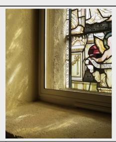
3 Secondary glazing was added to the windows, improving energy efficiency.
