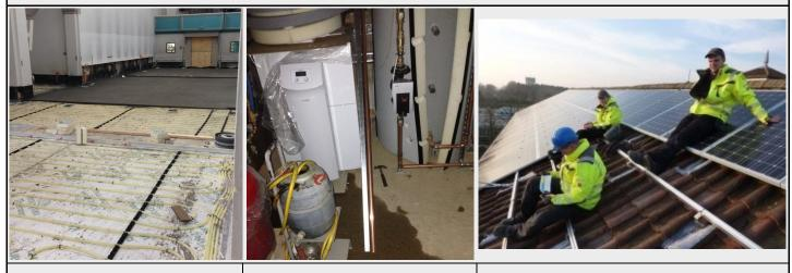
I New pipes were laid under the floor, which was also fitted with insulating material. 2 The ground source heat pump runs on electricity to draw heat from below ground and into two buffer tanks. 3 Solar PV panels generate more than enough electricity for the new heating system, meaning the surplus can be sold and provides a modest income stream.
