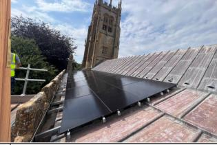
3 Solar panels were fitted to a special mounting system to prevent damage to the lead roof.
