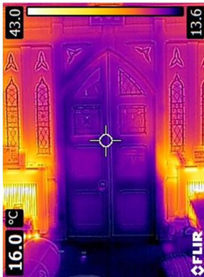
Below: Thermal image showing heat loss from cold air coming under a church door.
