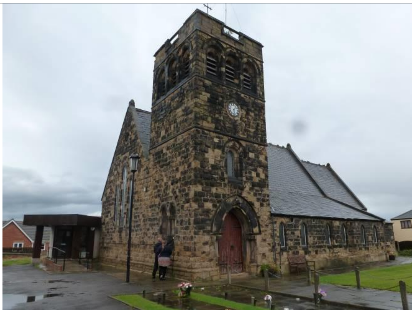
Exterior view from South
