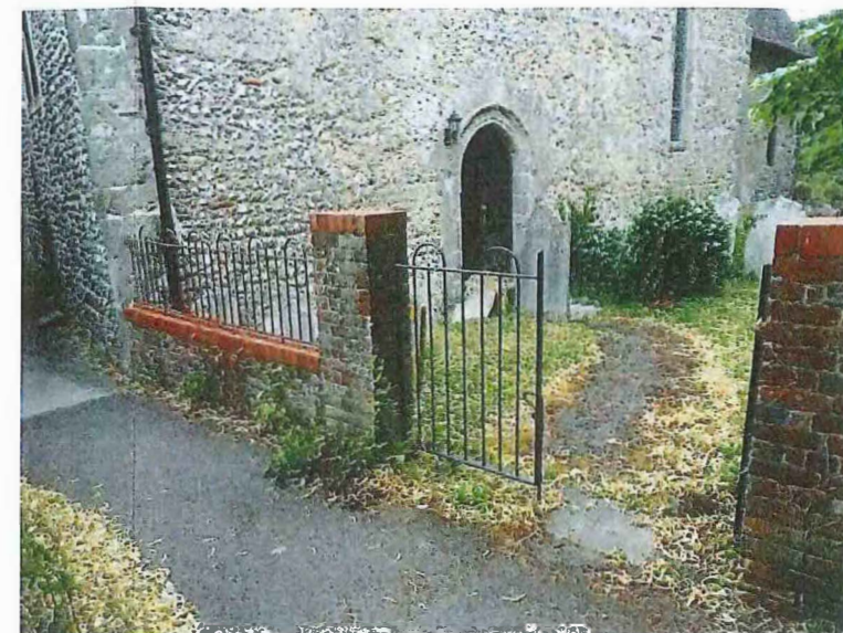
Fig 1 View of footpath from the back pavement to the south door of The Old Church.
